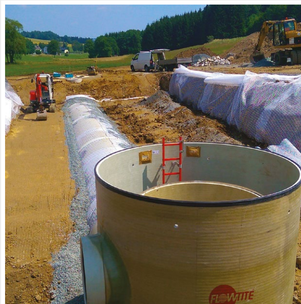
Stormwater overflow, trough inlet
