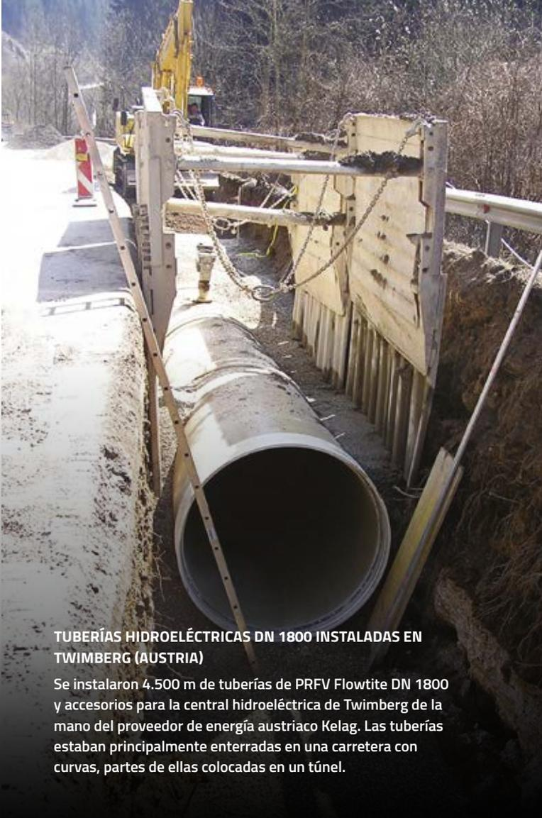
**TUBERÍAS HIDROELÉCTRICAS DN 1800 INSTALADAS EN TWIMBERG (AUSTRIA)**
